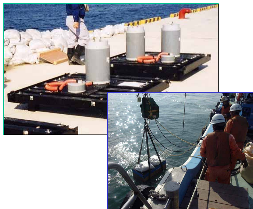
Photo: Installation of sensor
